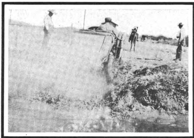
Traction was difficult in such spots on the way
